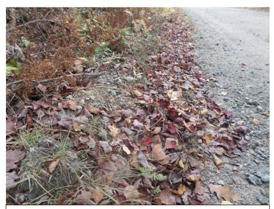
Road shoulders and ditches are misshaped, preventing water from reaching the ditch or moving effectively. Poor crown and grader berms also cause water to run along the road, picking up sediment before entering a wetland in segment 122739.
